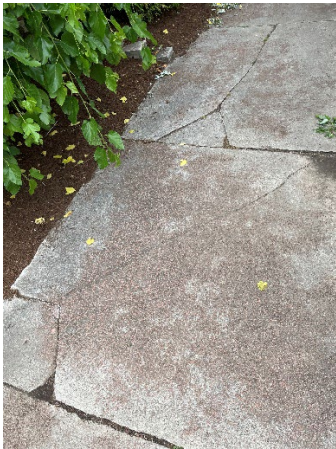
4) Lindell Blvd (between Whittier and S Sarah)- one section w deep cracks, other bad section aren't on the walkway but on adjacent sections leading to the road
